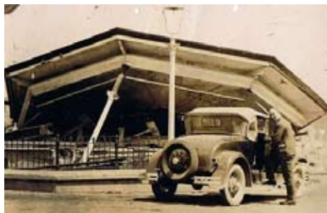
Collapsed Band Rotunda, Napier, 1931.
